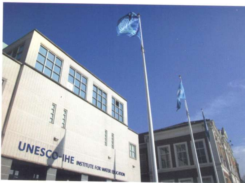
Figure 17. The UNESCO-IHE building in Delft, the Netherlands
